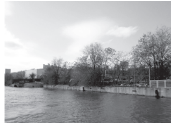
Fig. 37: Existing conditions at the proposed Fitness & Play site
